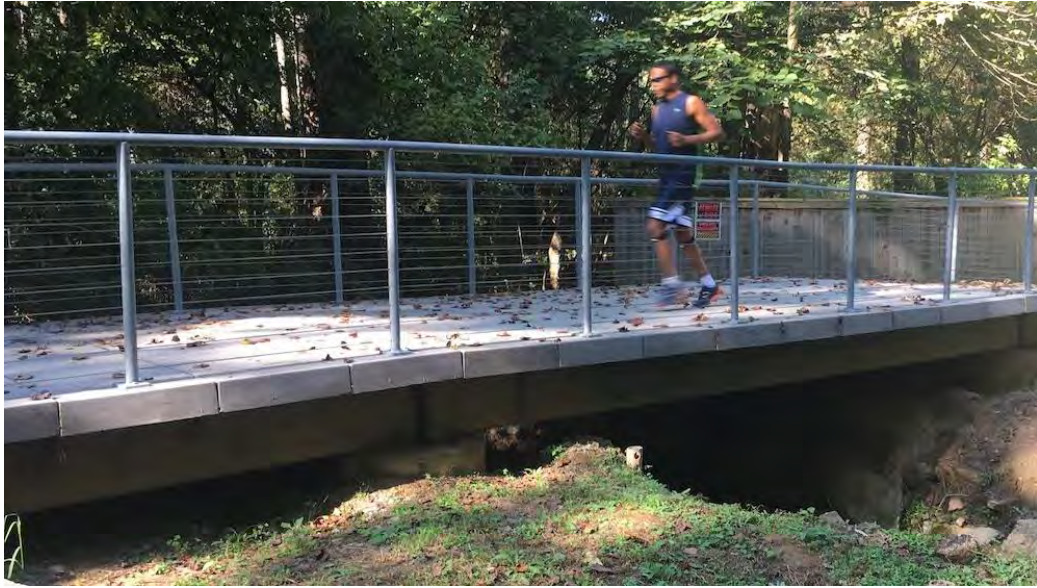
Fig. 8 – Example of an Engineered Path and Stream Feature
